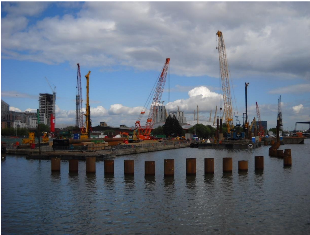
Fig. 1. An example of a development in the Tower Hamlets area at Canary Wharf. The dock is being modified in advance of construction. The development will require large quantities of aggregates; to fill the dock and in the manufacture of concrete.
