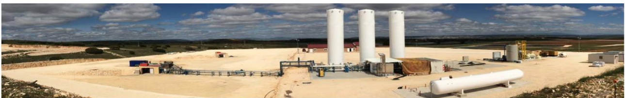
Hontomín Technology Development Plant, Northern Spain
